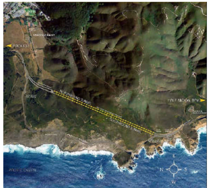
Aerial View of Tunnel
