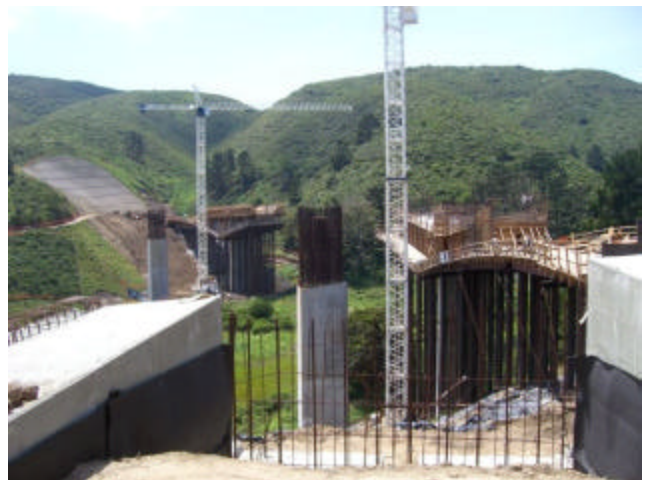
Bridge Under Construction; View to South
