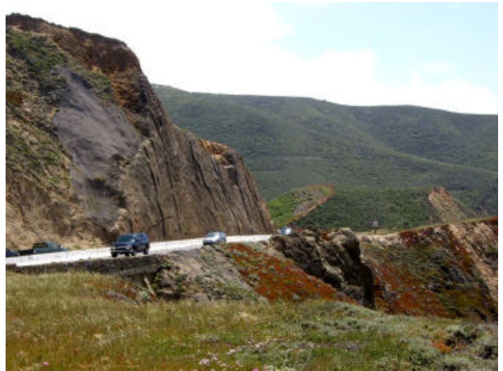
Fake Rock Wall at Southern Approach to Tunnels; View to South
