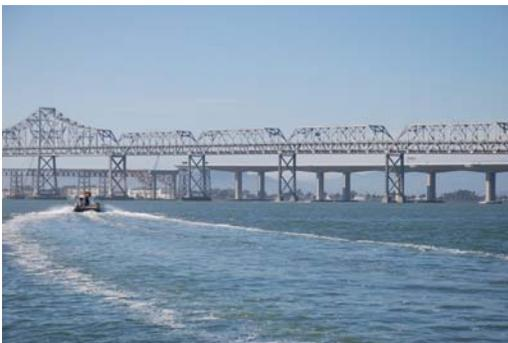
New bridge construction from Yerba Buena to the Oakland “touchdown” is being done because of the significant damage that happened to the old bridge during the LPE. Although the old bridge was designed to be useable for 150 years, its rigid design and substandard seismic elements make it
