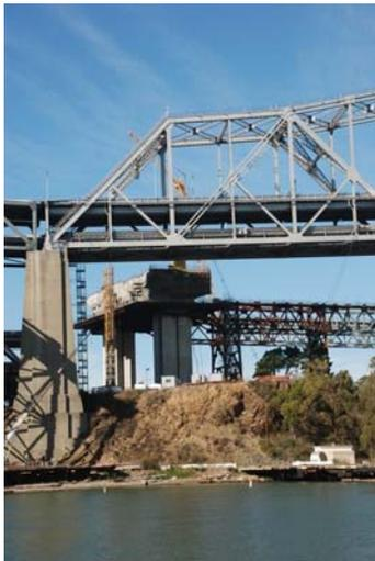
*With the old / existing bridge in the foreground, the W2 pier can be seen in the background along with a portion of the temporary scaffolding that is used to slide the new road sections in to place. The bedrock in the foreground was conclusively determined to be our outcrop for the day.*
