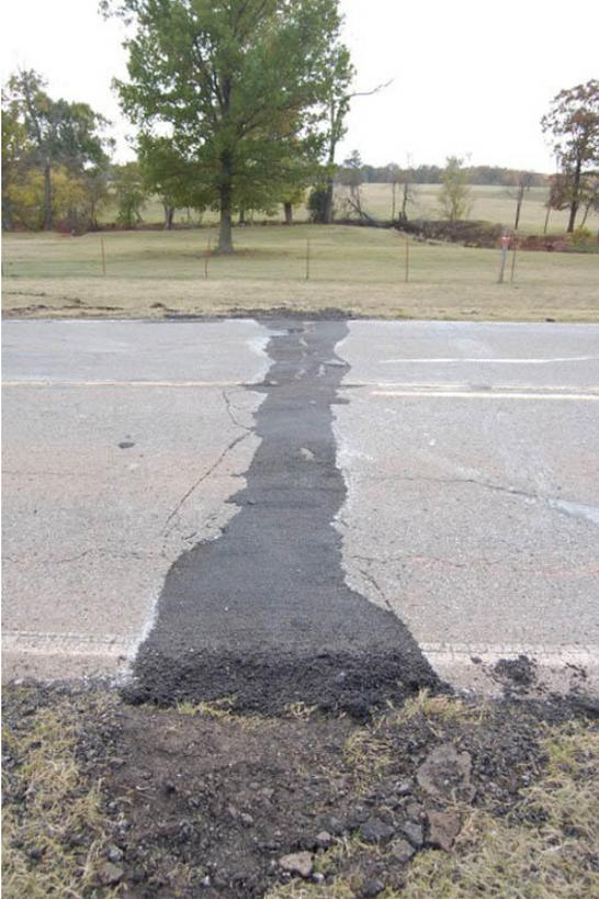
*A 2011 magnitude 5.7 quake near Prague, Okla., apparently triggered by wastewater injection, buckled U.S. Highway 62. (Credit: John Leeman)*
