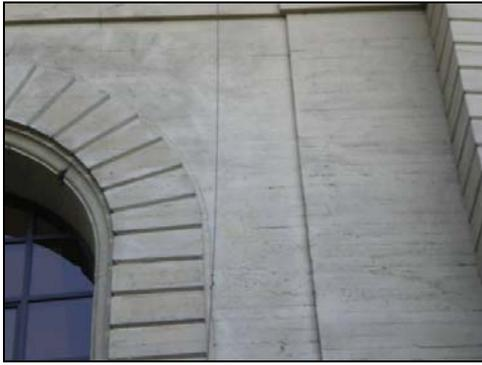
**Figure 3 Tension cracks on the side of the Berkeley Memorial Stadium north entrance.**
