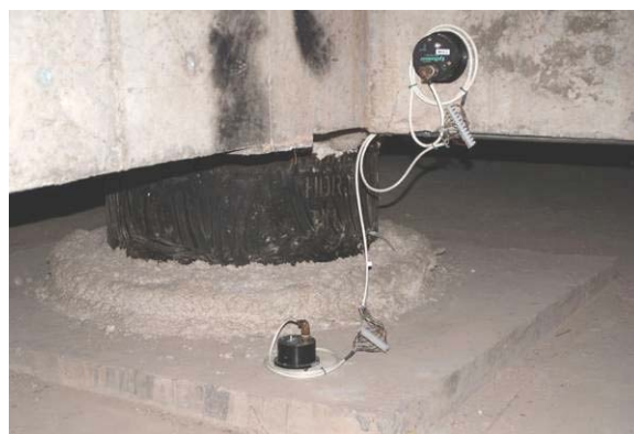
Figure 8 Base isolator cushion and accelerometers underneath the Hearst Mining Building.
