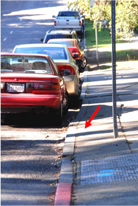
Figure 7 Curb offset on Dwight Way looking downhill (west). Red arrow notes general vicinity of creep offset on the Hayward Fault.
